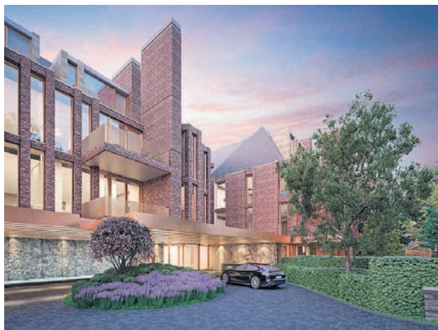
No. 7 Dale uses Algonquin limestone on its facade and solid bronze pickets on the north balconies, which will age into a rich patina over time. The building also features Kolumba bricks at the building's base. IMAGE COURTESY OF PLATINUM VISTA
